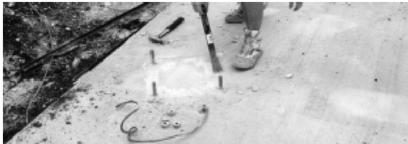
Figure 1-3: Scraping Foundation Pads
